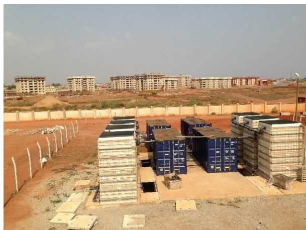
SATURN system 7,500 PE system in Ghana. The system cleans wastewater from the apartment buildings seen in the background.
