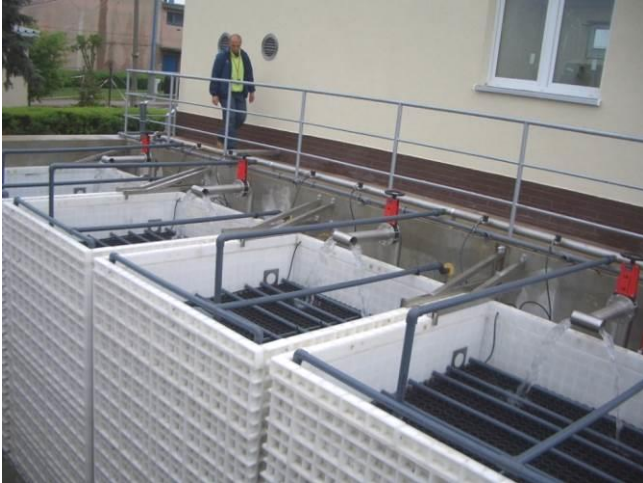
BioReactor system under installation in on site built concrete tanks
