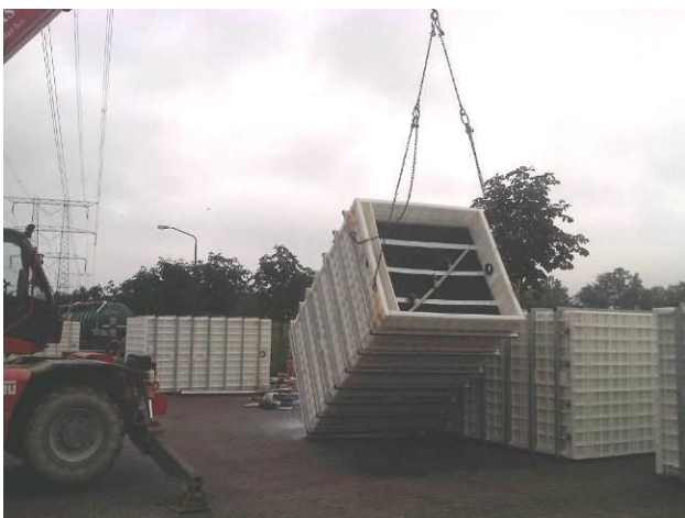
BioKube cleaning unit under installation in Holland. Each unit will clean 150 m3 wastewater pr. day
