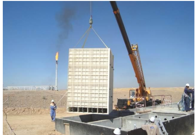
BioReactor cleaning units are delivered ready to install in 20 or 40 feet containers. Typical time for installation 1 – 5 days before system operational.
