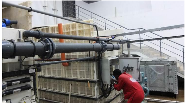
Treated water to be reused so system equipped with UV lighting. Easy access for maintenance and service.
