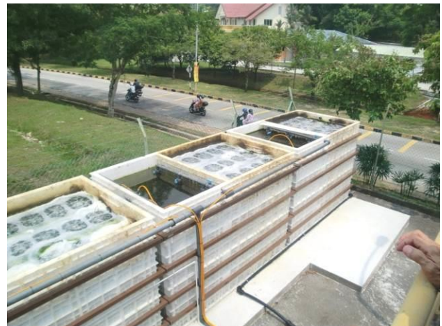
Jupiter system in operation at University in Kuala Lumpur, Malaysia. Installed above ground. Note the even distribution of the aeration.
