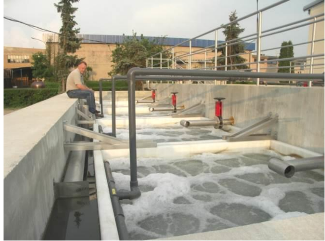
BioReactor system in operation. Notice the very even distribution of the aeration.
