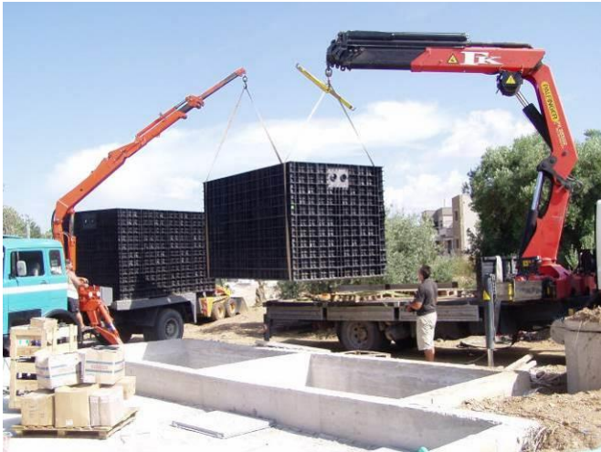
Jupiter 75 system under installation.
