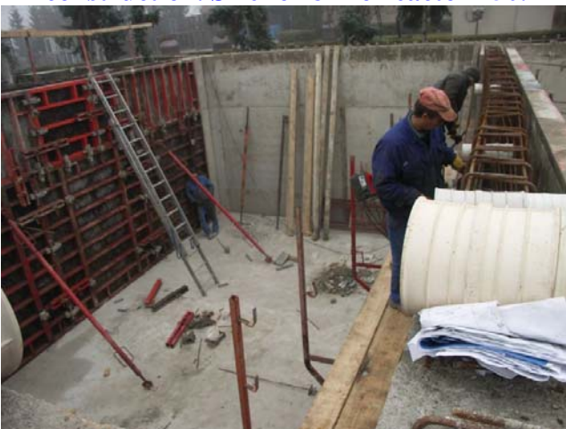
Concrete tanks for vegetable factory under construction. Size for 8 BioReactor 150.
