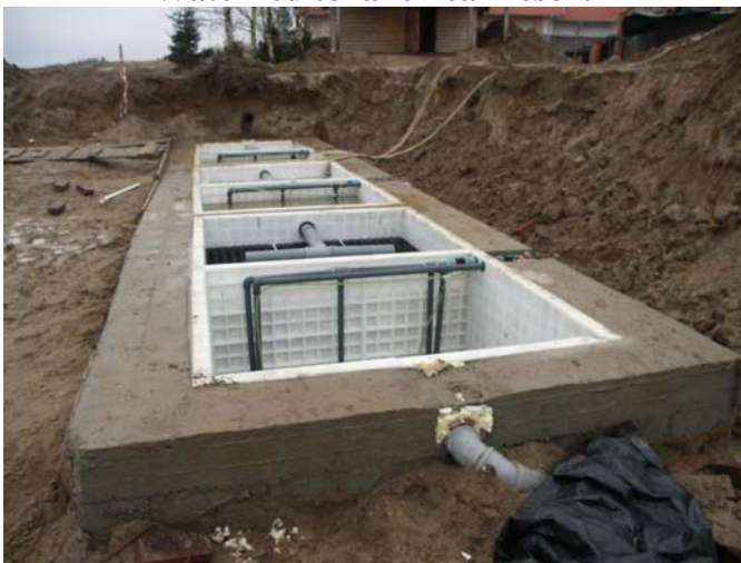
Resort Hotel, Brodnica, Poland under construction 50 m3 / day (300 PE) Water led to lake near resort
