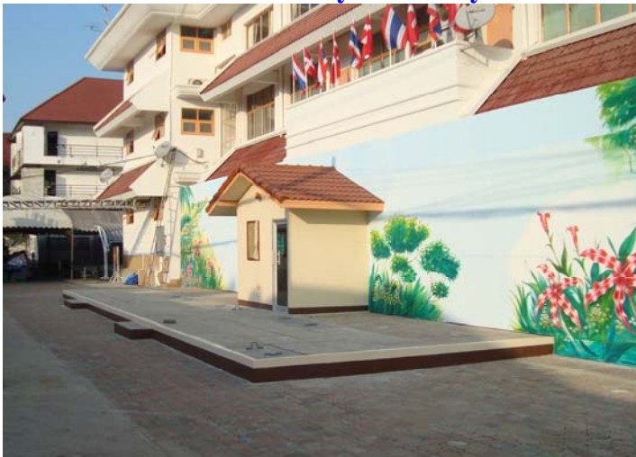
Town Hall Notamburi, Bangkok, Thailand. 75 m3 / day (400 PE) Cleaned water is recycled to city lake.
